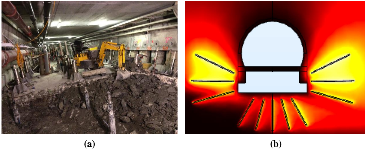
Figure 2 (a) Extreme floor heave in a Swiss tunnel; and (b) temperature field around a tunnel with thermal control of swelling
