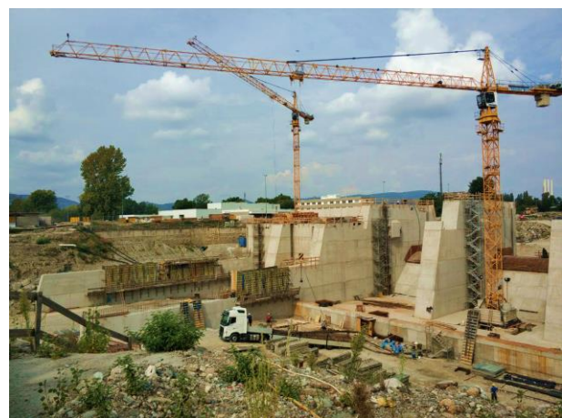
Figure 2. Site visit for a project "Murkraftwerk Graz"
