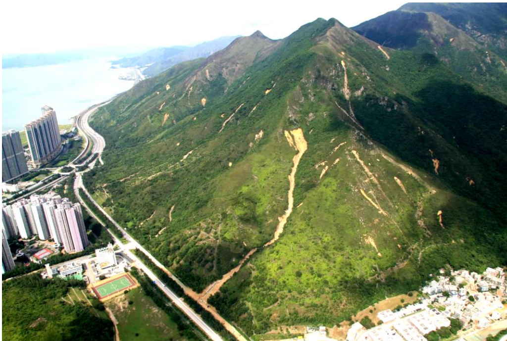
Cheung Tung Road Landslide, Lantau Island, Hong Kong
