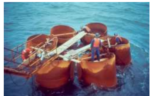
Construction of large diameter battered drilled concrete shafts for approach spans (1994-1995).
