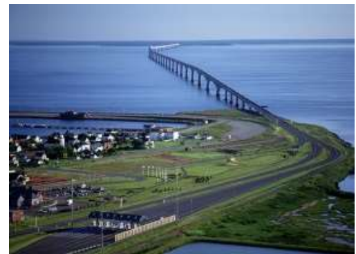
After completion of construction (1998).
