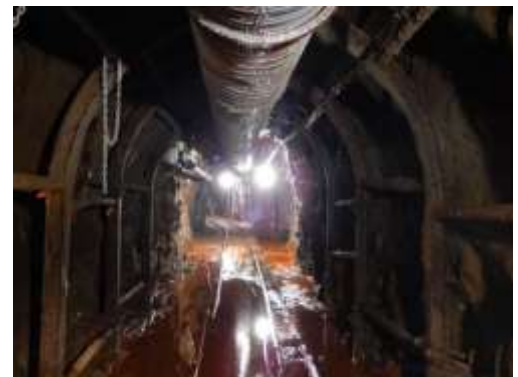
Typical conventional drill and blast, horseshoe-shaped, extensively supported adit
