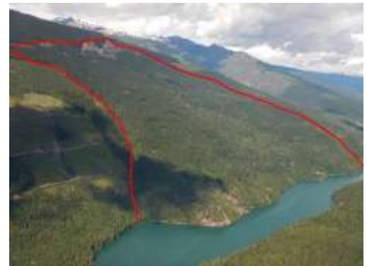
Aerial view of Downie Slide (outlined in red) looking up the Revelstoke Reservoir and Columbia River valley.
