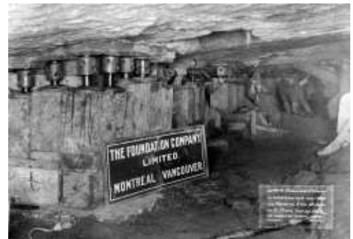
Shoring screws used to lift structure.
