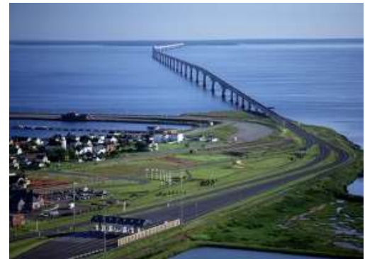
After completion of construction (1998).
