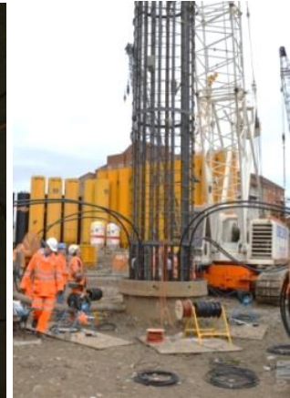
Fiber optics installation in energy piles
