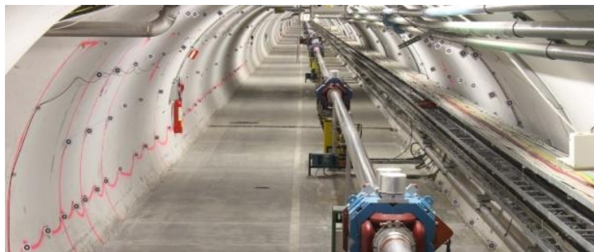
Long-term performance of CERN tunnels, Switzerland
