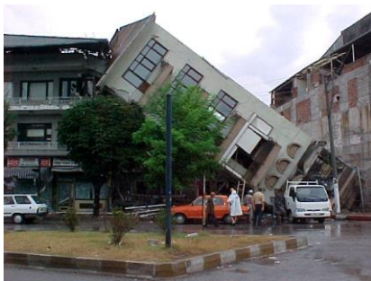
Tilted building due to liquefaction
