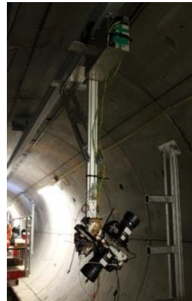
Computer vision for tunnel inspection
