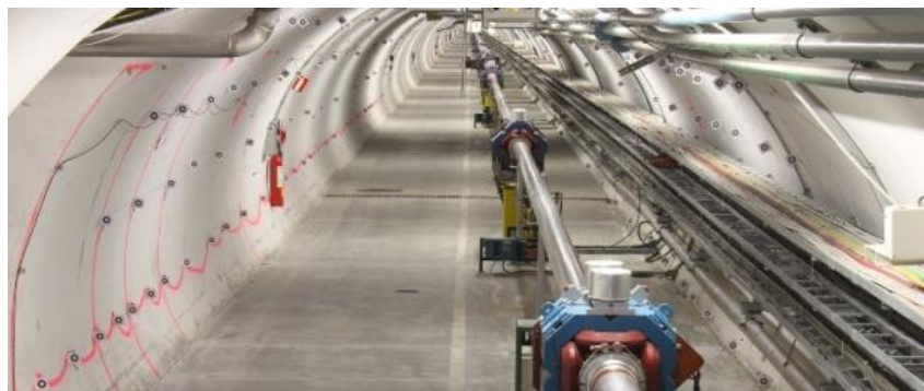
Long-term performance of CERN tunnels, Switzerland
