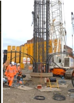
Fiber optics installation in energy piles
