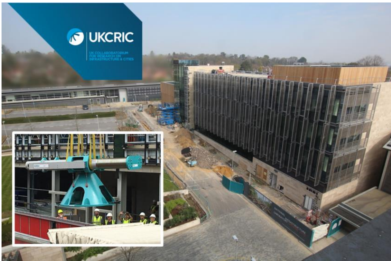
Figure 2. The National Infrastructure Laboratory at the University of Southampton. Inset: Delivery of the Actidyn C67-4 geotechnical centrifuge
